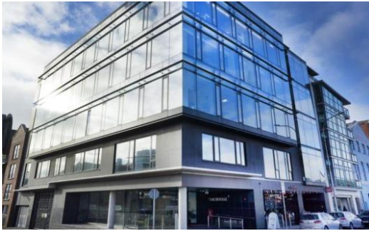
The Anchorage Building, Sir John Rogerson's Quay, Dublin 2
